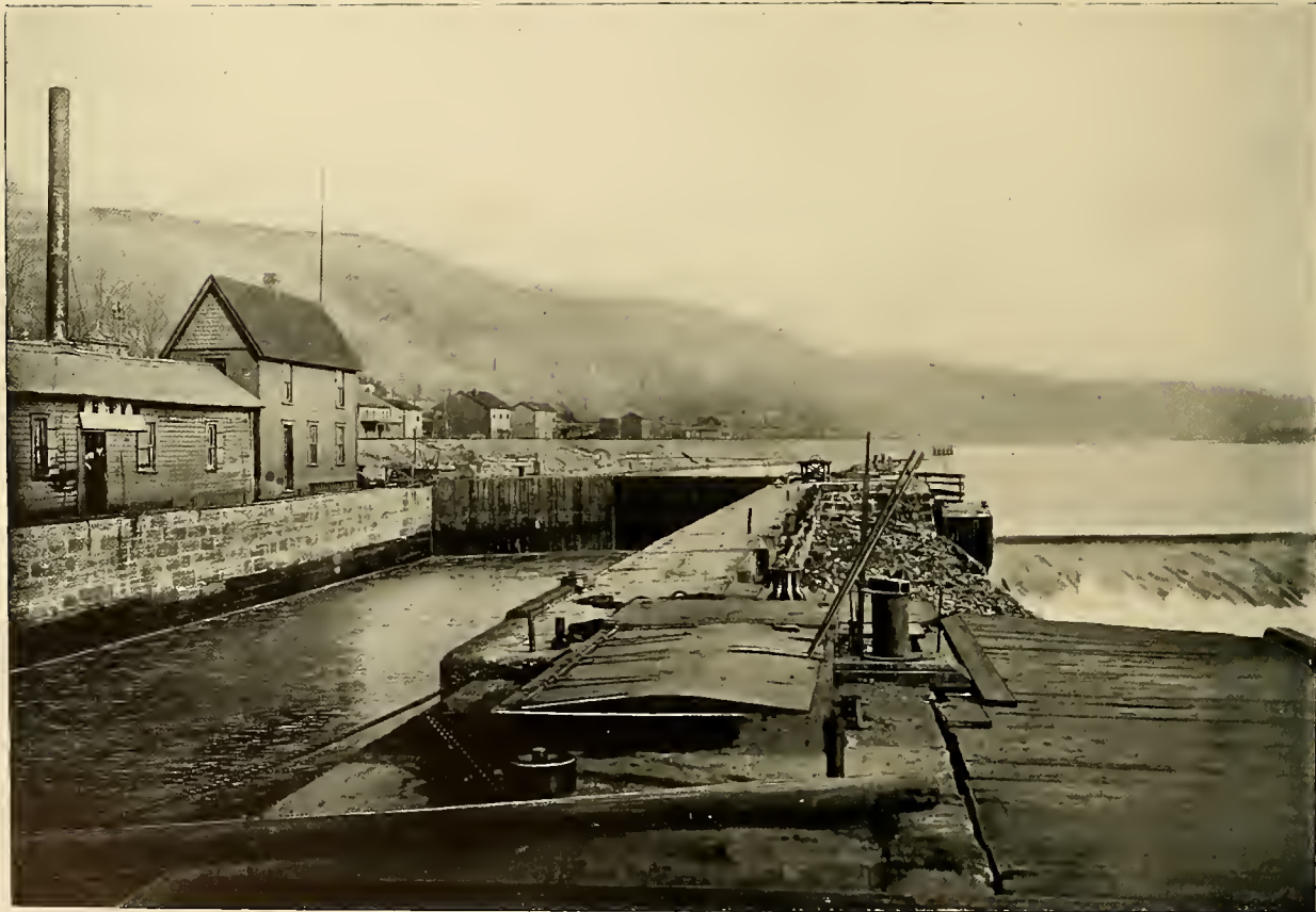
Lock No. 2, Monongahela River.
